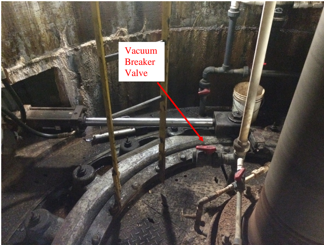
PHOTO 3-1 PIPING FOR VACUUM BREAKERS IN HEADCOVER
