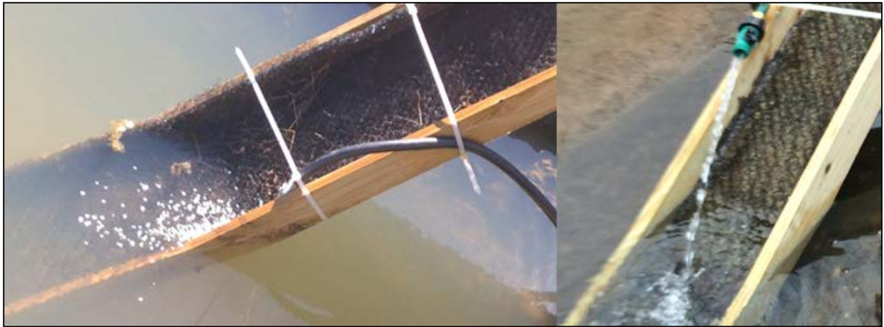
PHOTO 5 EXAMPLES OF ATTRACTION FLOW AT THE BASE OF RAMPS
