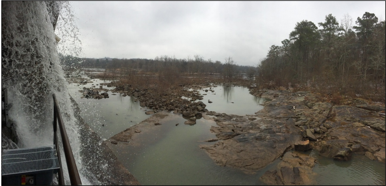
PHOTO 1 LEAKAGE FLOW AND COLLECTION BUCKETS USED TO PROVIDE WATER TO WEST CHANNEL ELVER TRAPS
