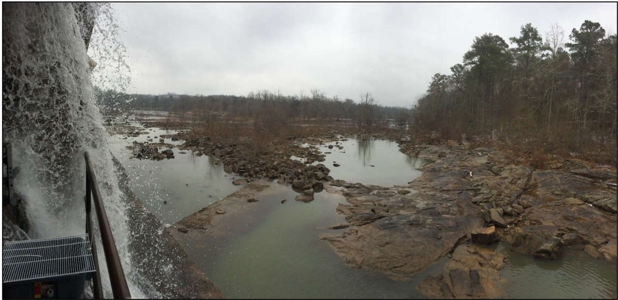
PHOTO 1 LEAKAGE FLOW AND COLLECTION BUCKETS USED TO PROVIDE WATER TO WEST CHANNEL ELVER TRAPS
