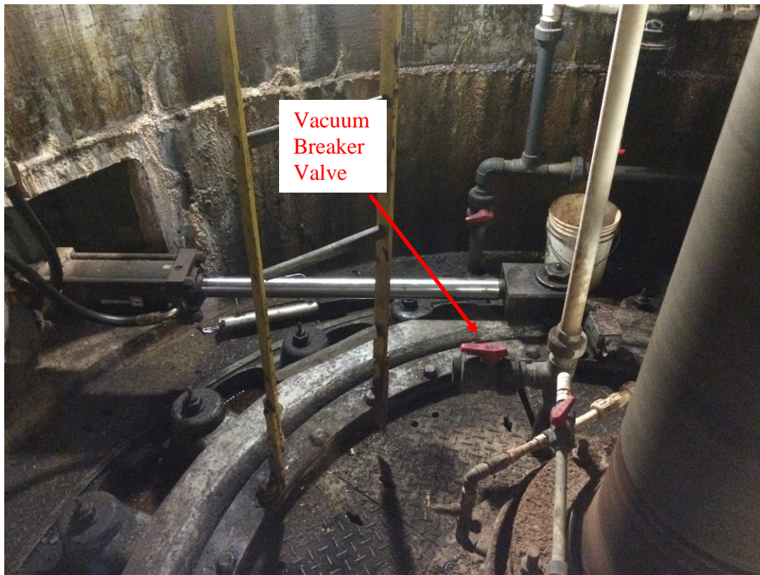
PHOTO 3-1 PIPING FOR VACUUM BREAKERS IN HEADCOVER
